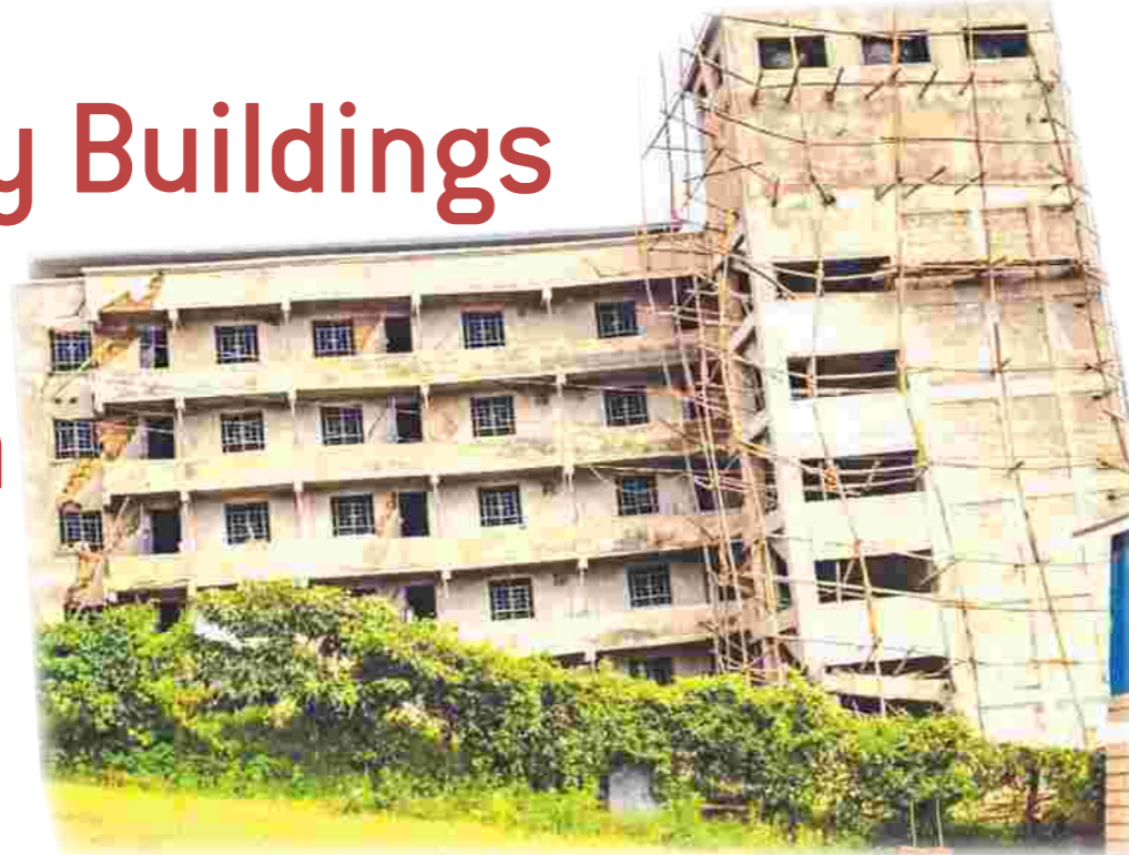
The building that recently collapsed at Kinoo in Kiambu County.
